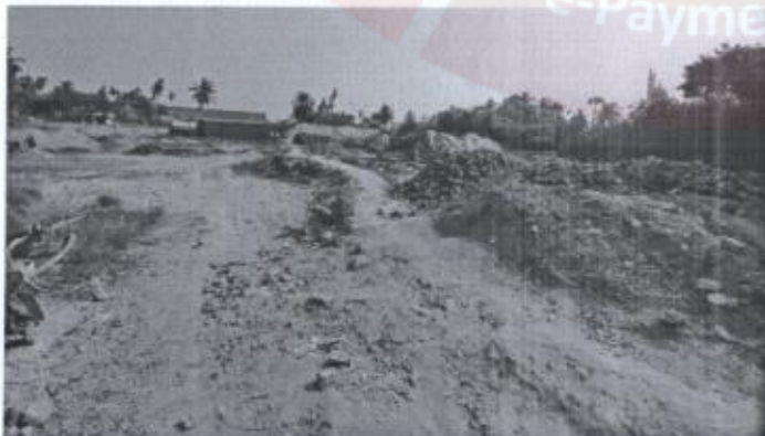
Figure 3: Status of site for construction of proposed 38 bungalows.
