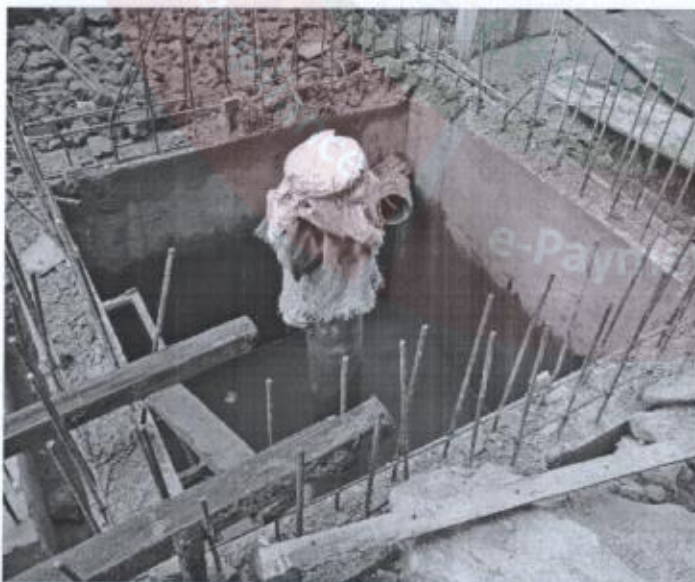
Figure 6: Construction of one of the rain water recharge pits.
